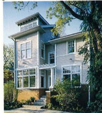
WILMETTE HOUSE: Addition at rear.
