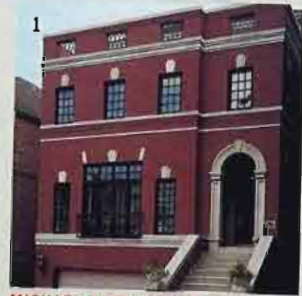
1 MICHAEL HERSHENSON Michael Hershenson Architects
