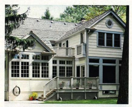
The remodeling affected the rear of the house (above). The left side was bumped out for the kitchen's breakfast area. The screen porch, library (left), and master suite occupy the area on the right. The shaded areas on the plans (below) indicate reworked or added space.
