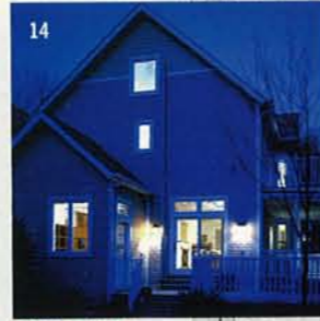
14 FOSTER DALE Foster Dale Architects
