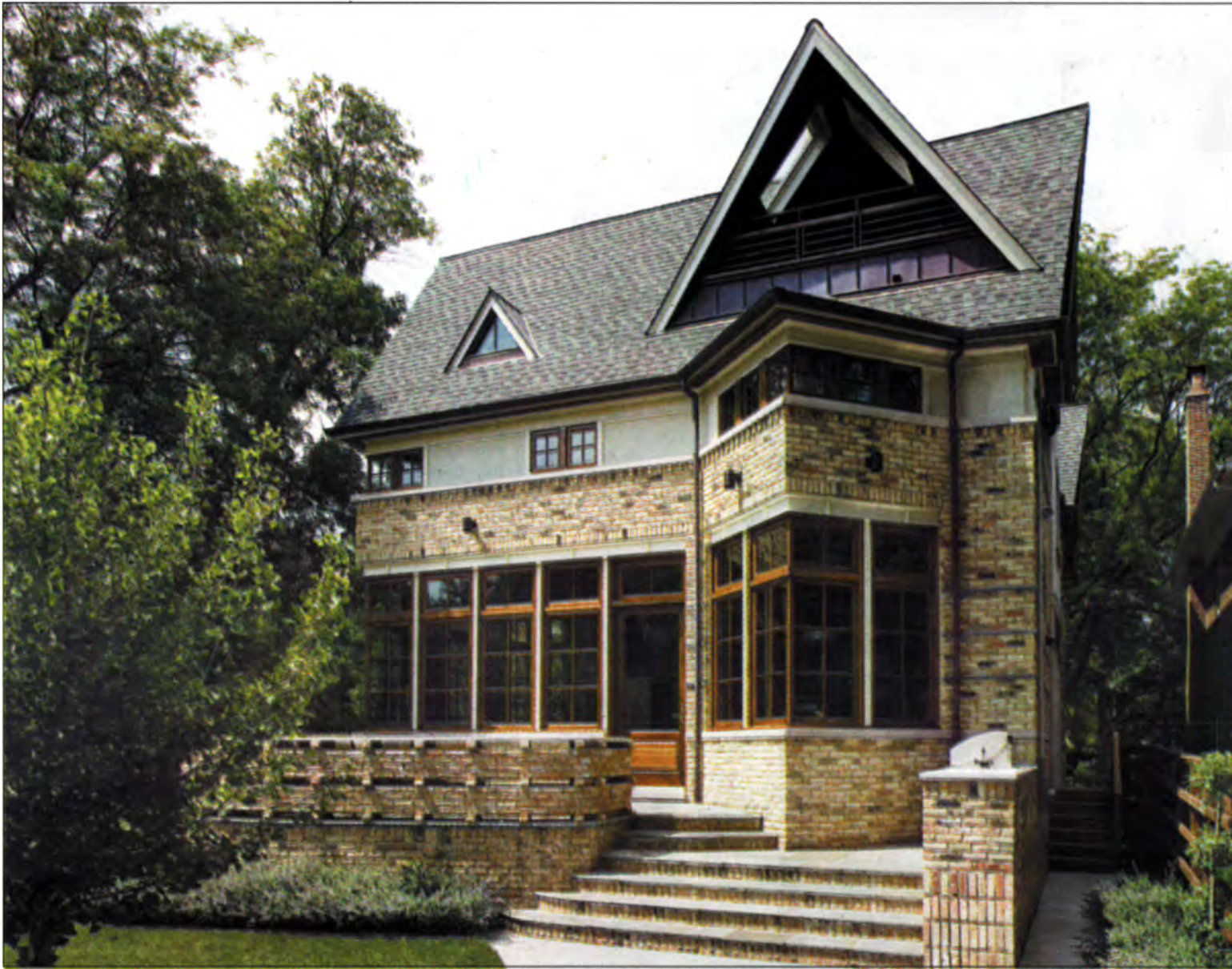
The exterior of Elissa Morgante and Fred Wilson's home marries Chicago common brick with other local materials, such as Indiana limestone and Douglas fir. JON MILLER/HEDRICHBLESSING PHOTOS
